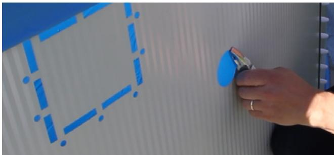
There are perforations in the pool wall for making holes for the skimmer and return tube. The holes can be cut out and all uneven surfaces are then removed with a file. Lastly, the edges should be treated with an anti-corrosion agent. If this is not done, the edge may rust.
